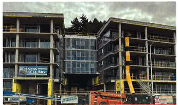
August 31st, 2021 construction progress
