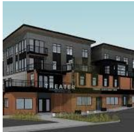
Theatre Nearing Completion
